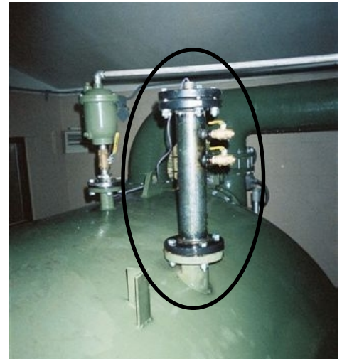
EPA 2000 - Pressure Filter Sensor Installation
