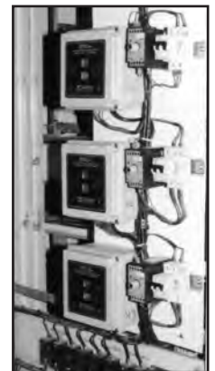
Also installed in a coal-fired power plant is the SFD-2 power supply/conditioner board with the optional fiberglass enclosure.
